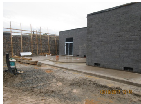
Energy centre with base for sprinkler tank now installed
