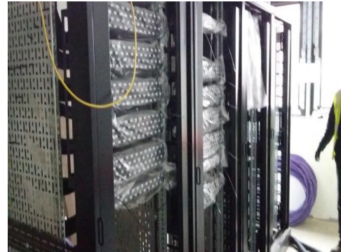
Data cabinets being installed on second floor
