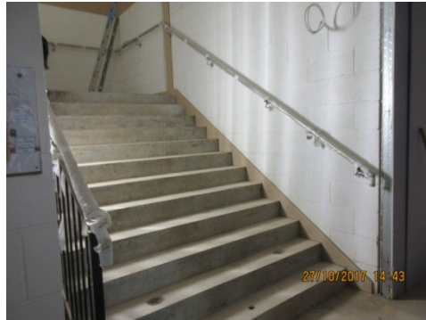
Stringer skirting being installed on stairs
