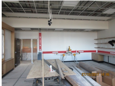
Fitted furniture being progressed on 2nd floor
